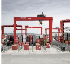
Automatic stacking crane
